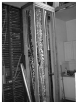
Space around Ducts may be a path
